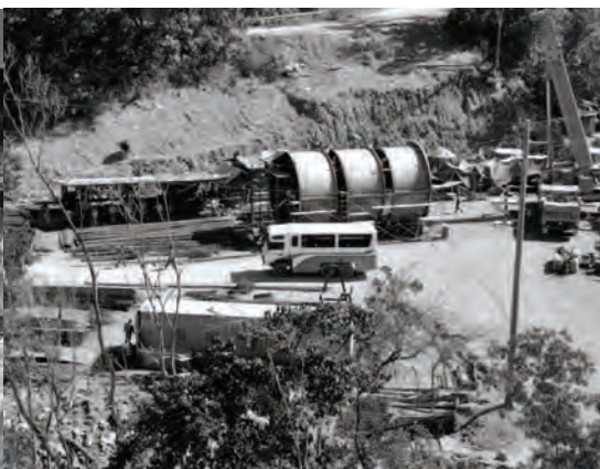
Assembling of new ball mills
