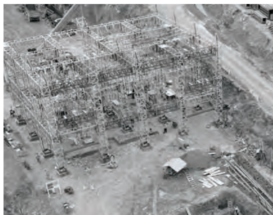
New power plant station
