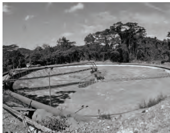
Tailings thickener no.7
