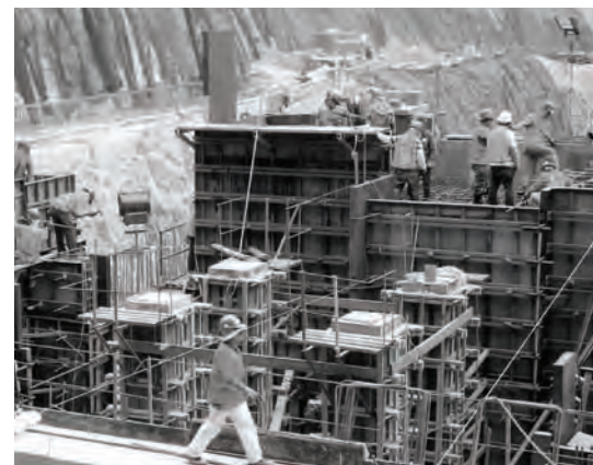
Concreting works at Primary Crusher Line 2
