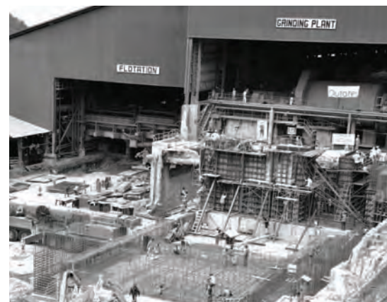
Construction of Ball Mill 8 and 9 areas
